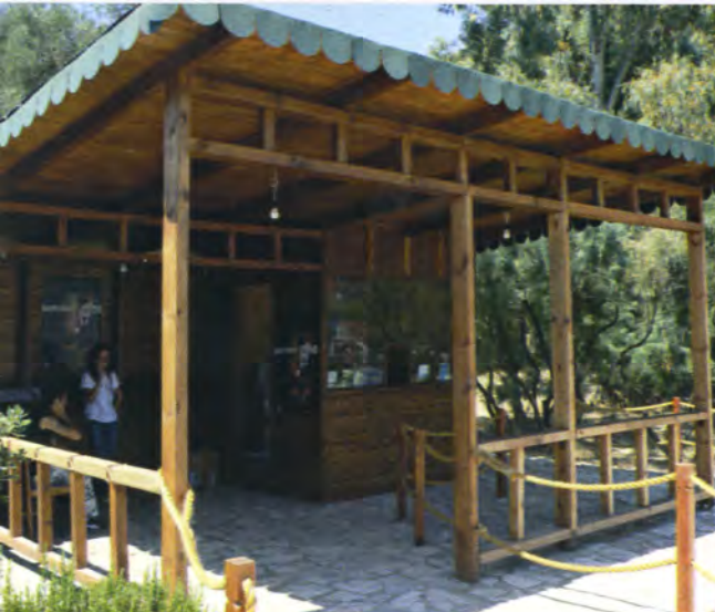
The new ticket office
