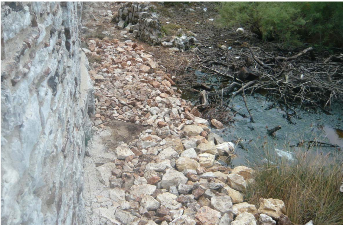
Backfilling of the ponds and continuation of the platform in sections 8.ga – 8.fa
