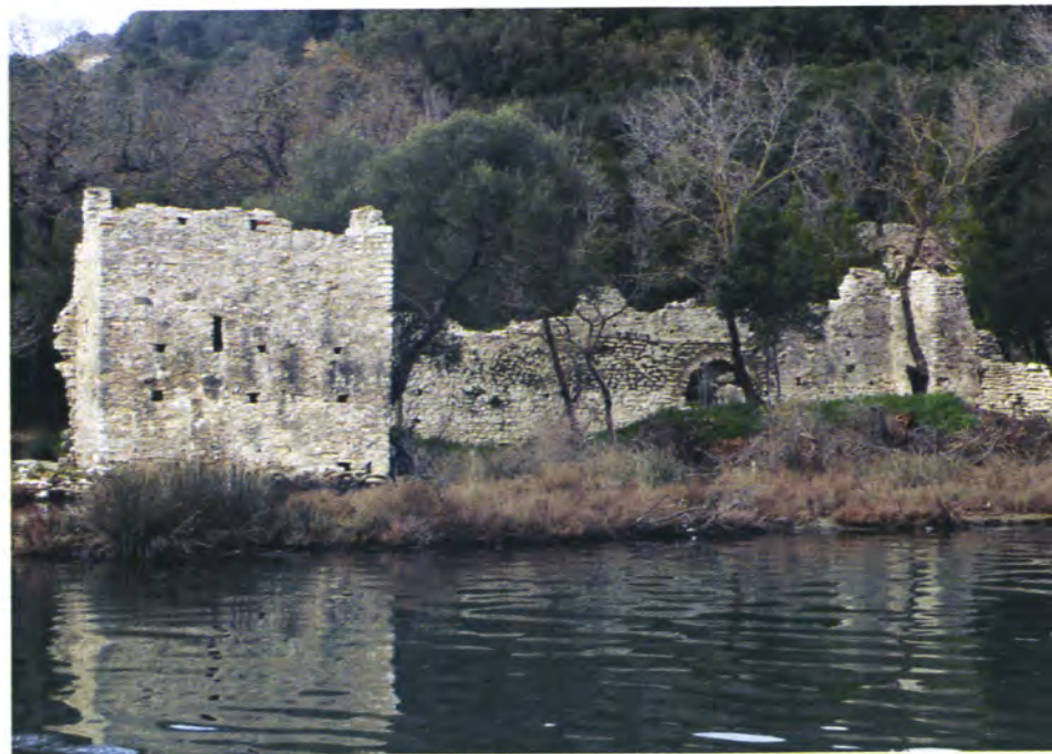
Water Gate and Tower after conservation
