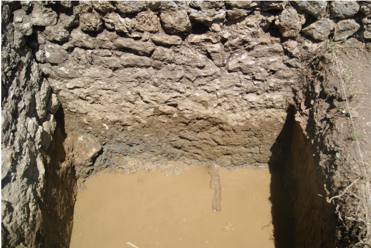
Fig. 13 View of foundation of the northeast curtain wall showing the wooden beam beneath the wall, Trench 3
