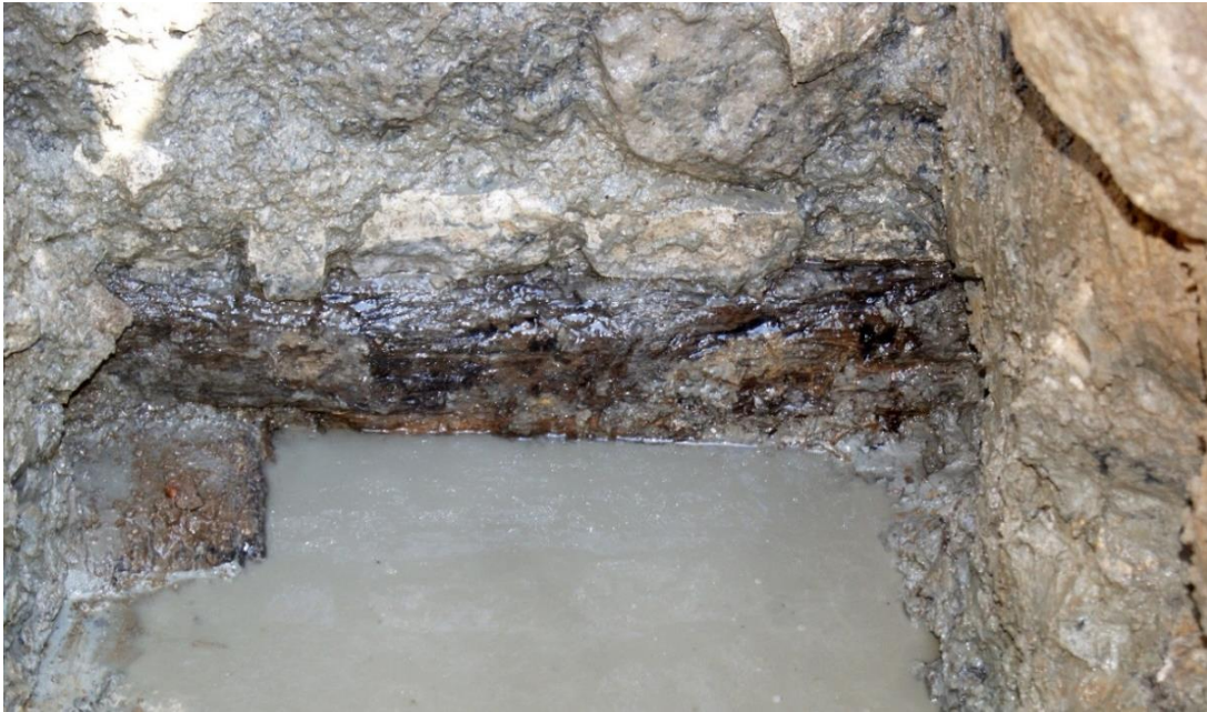
Fig. 10 showing beam cross placed on to which the southern curtain wall rises, trench 2
