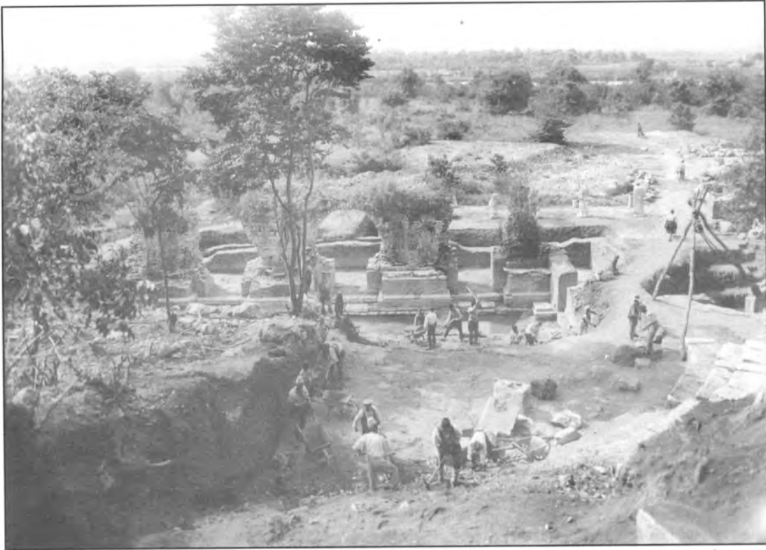
Excavation of the theatre at Butrint (Ugolini archive 1929)
