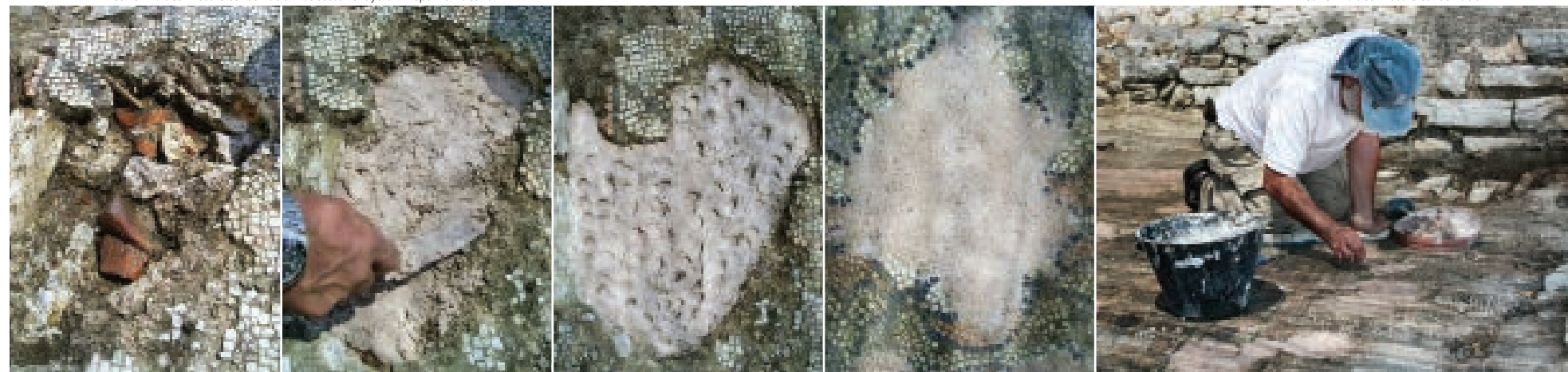
Triconch Palace mosaic conservation: successive layers in repair of lacuna
