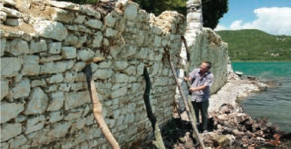
Butrint city walls with props supporting collapsing section prior to conservation
